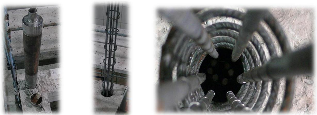
**Figure (2):** Installation of EDILINNOVA Pillar Bone Rehabilitation Technology for Existing Reinforced Concrete Building
